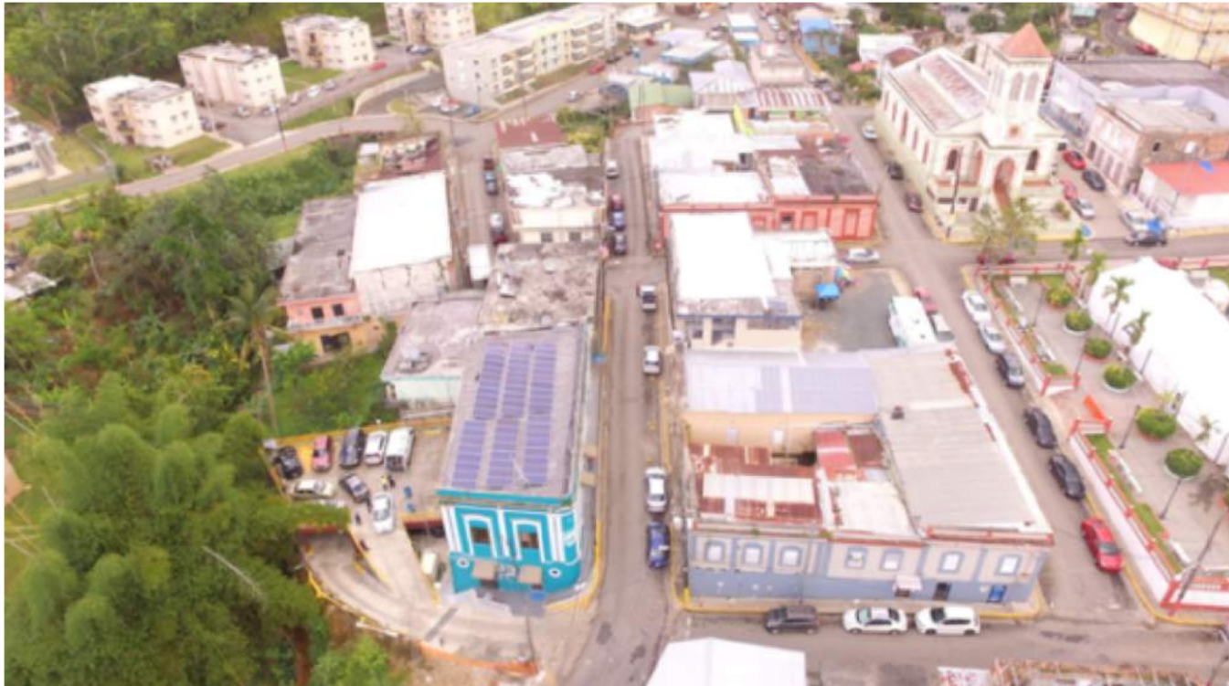
The completed 18 kW solar system at the Migrant Health Clinic in Maricao, Puerto Rico. Source: Kelsey Clark, The Solar Foundation
