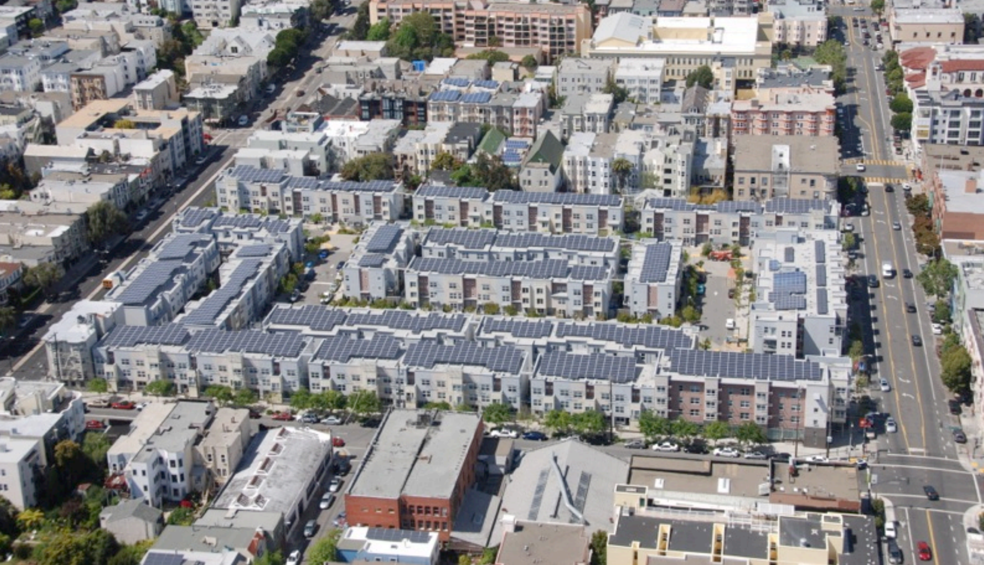
Ecoplexus project at the Valencia Gardens Apartments in SF. ~800 kW meeting ~80% of the total annual load.
