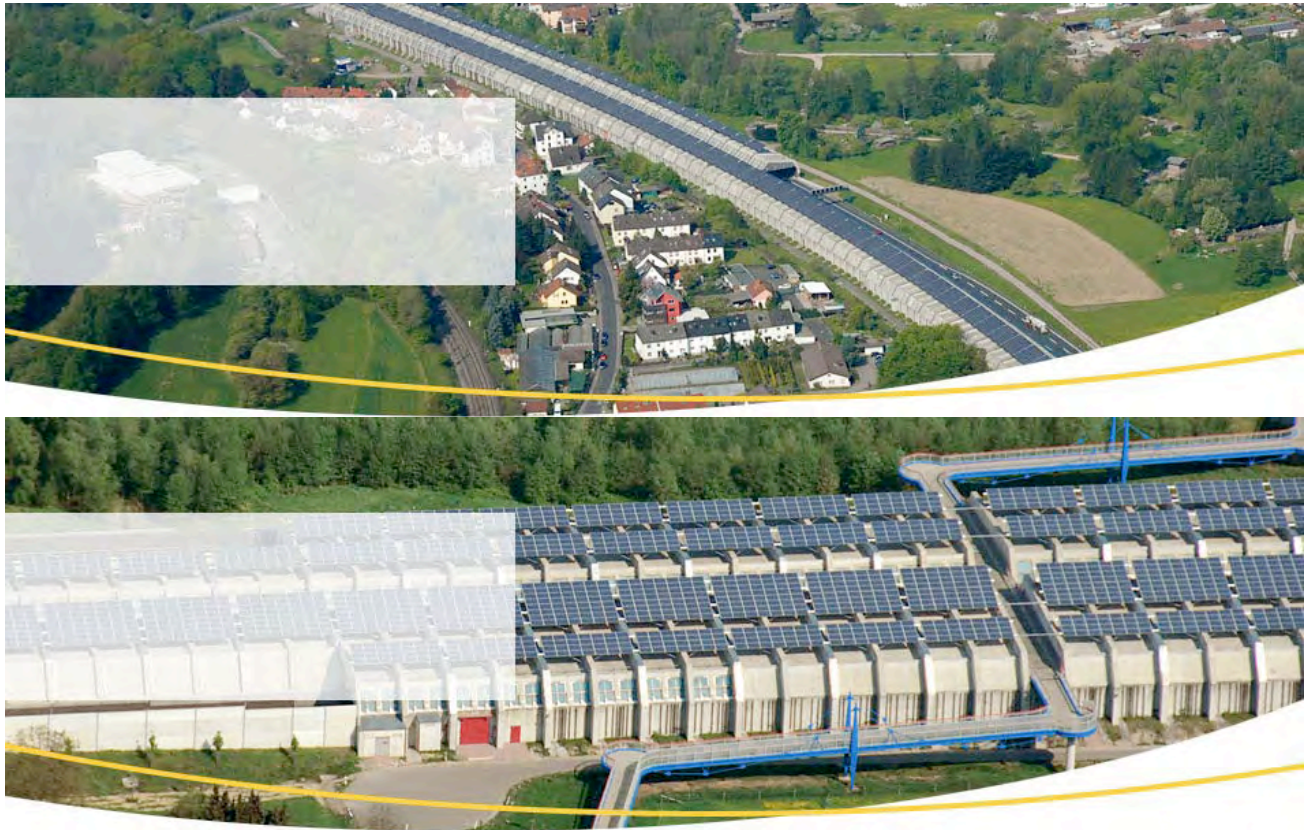
Figure 3: A Pioneering 1.6 MW Project for Enclosure of Transportation Noise on Highway A3 between Goldbach and Hösbach. 12
