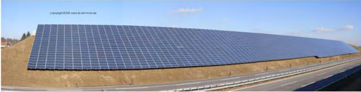
Figure 2: Example of Solar Power Installation at an Earthen Slope Used for Noise Abatement on Highway A96 (similar to the Freising Project)
