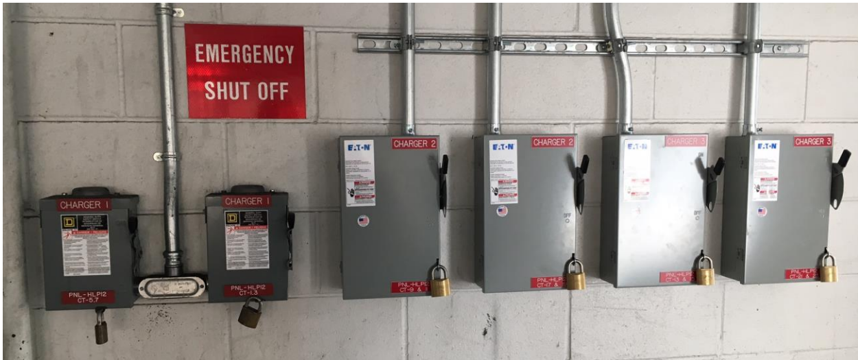
Figure 8: Additional Disconnect Switches Required by some EV Charger Codes
