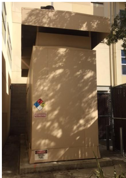
Figure 34: Existing diesel backup generator
