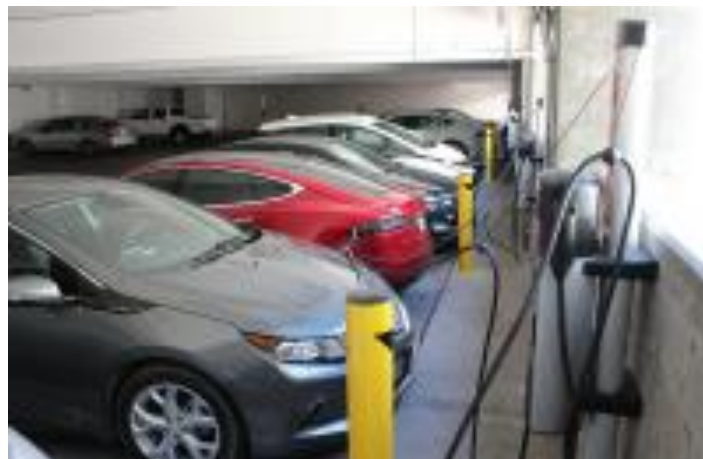
Figure 43: EV chargers in Bryant Street garage
