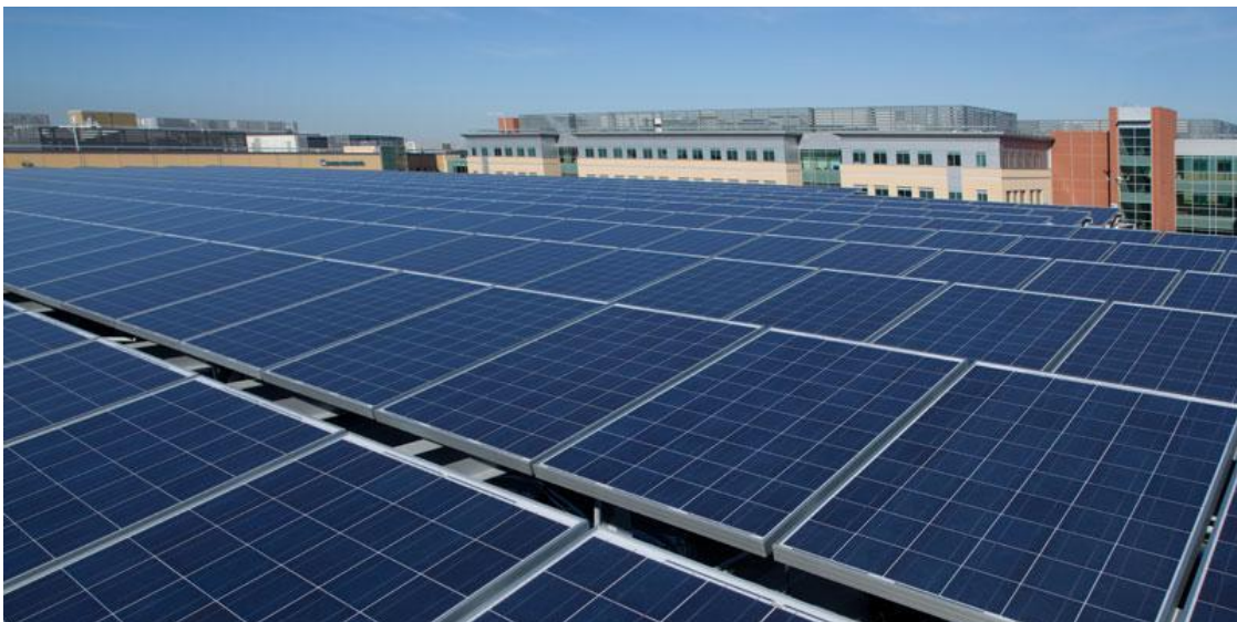
Figure 38: Solar panels cover parking structure in Santa Clara
