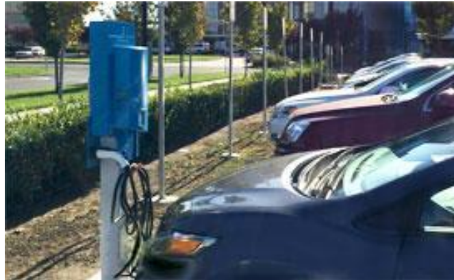
Figure 39: EV charging station in Vacaville, CA
