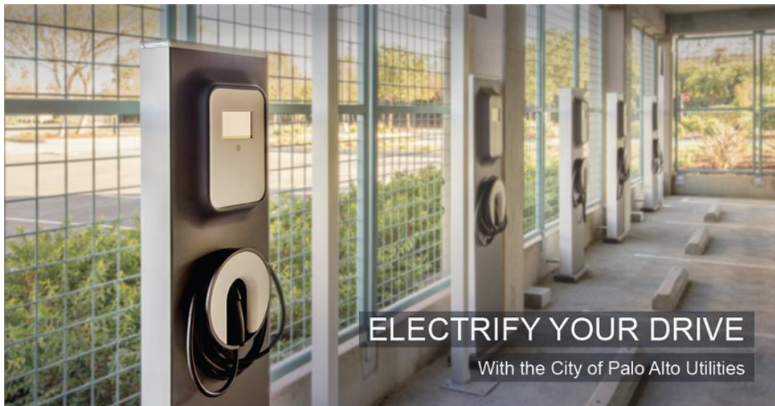
Figure 44: Electric vehicle chargers at City of Palo Alto
