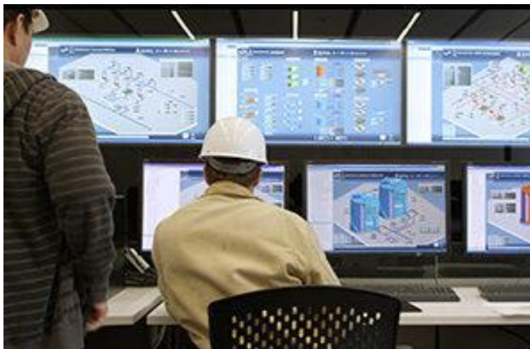
Figure 26: Central Energy Facility Control Room
