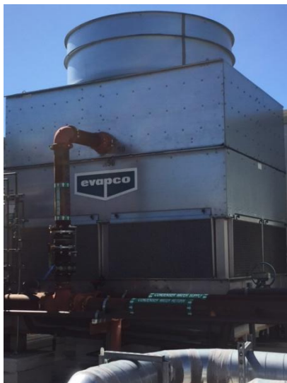
Evaporative Cooling Tower
