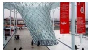
Milan trade fair to commission world's biggest rooftop solar power installation
