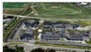
Google to build largest US Corporate Solar Installation
