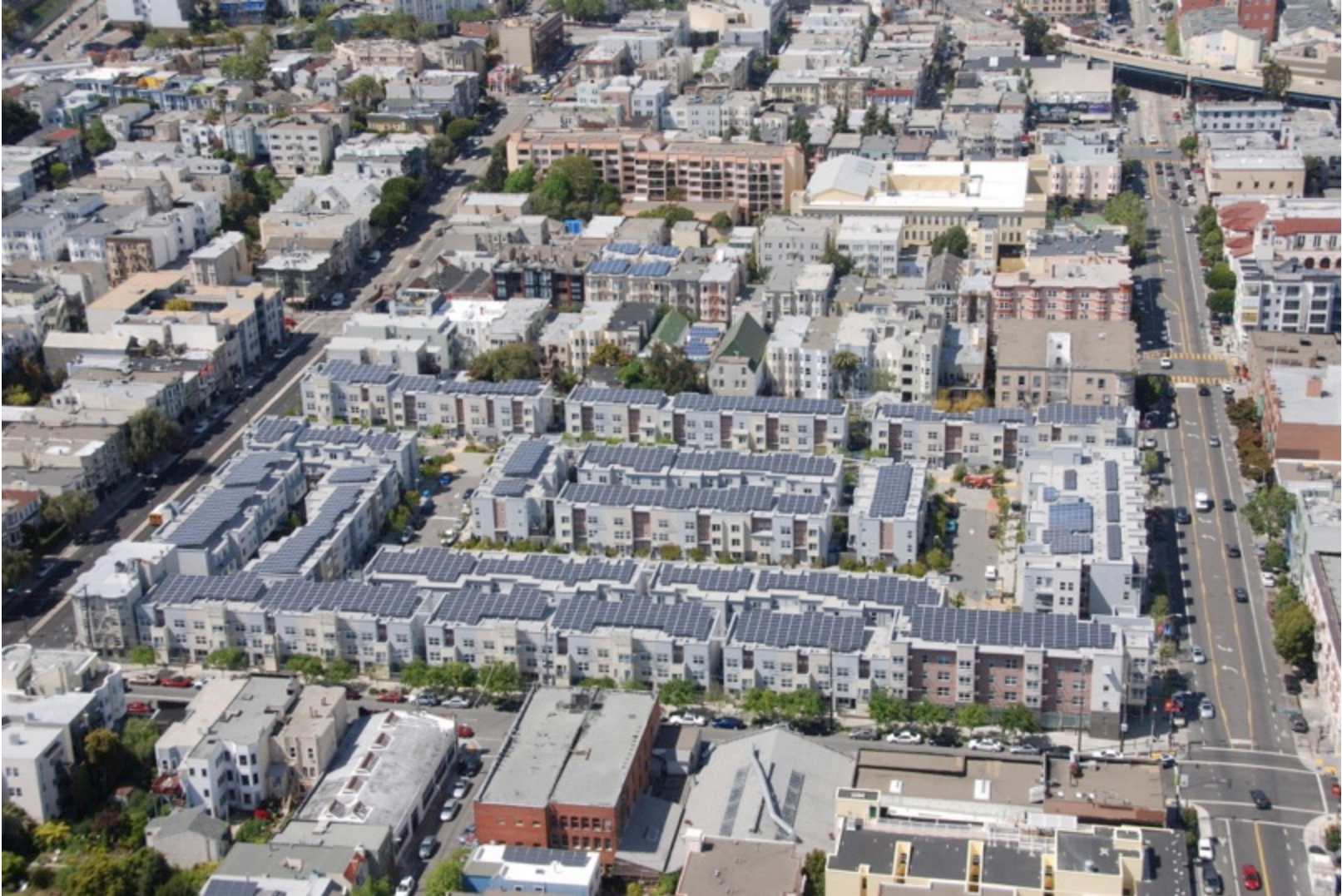
Ecoplexus project at the Valencia Gardens Apartments in SF. ~800 kW serving ~80% of the total annual load.
