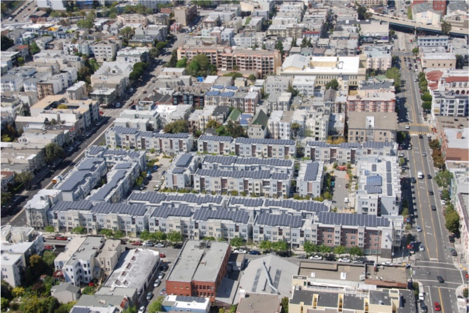
Ecoplexus project at the Valencia Gardens Apartments in SF. ~800 kW serving ~80% of the total annual load.
