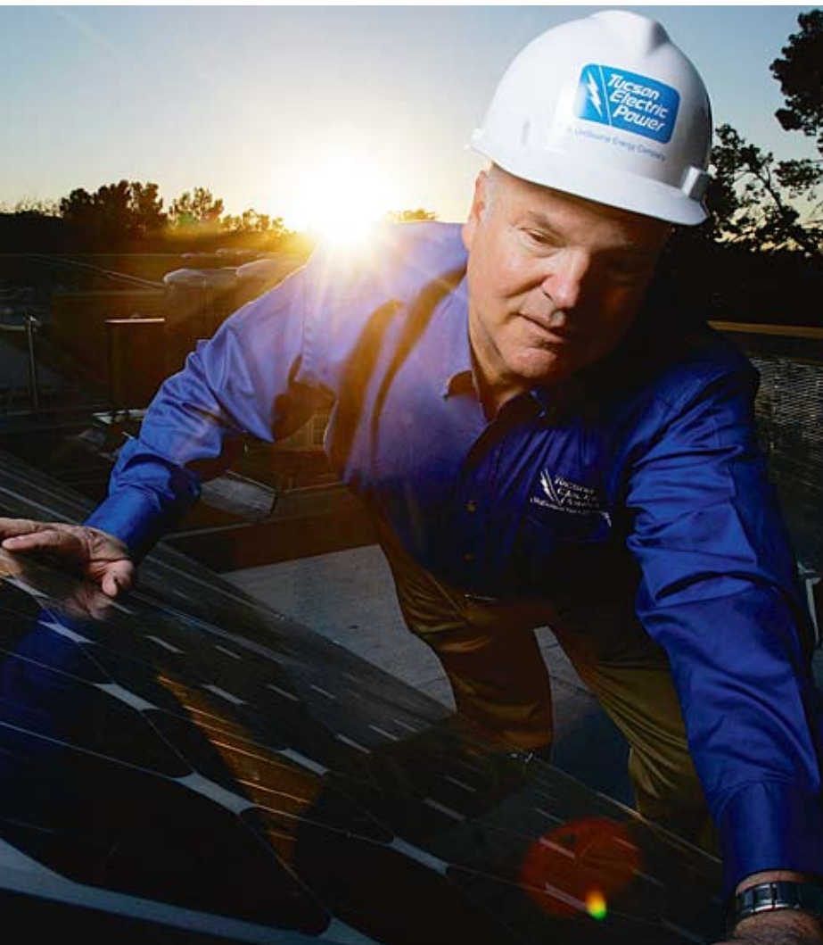
One of the TEP employees inspecting a solar installation at Tucson's Reid Park Zoo.
