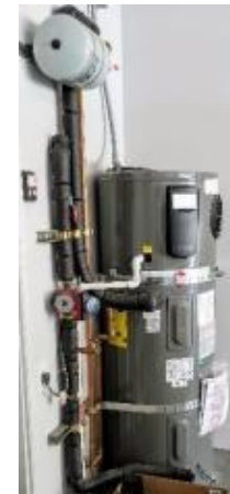
H.P. water heater
