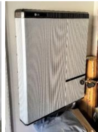
L.G. Chem energy storage
