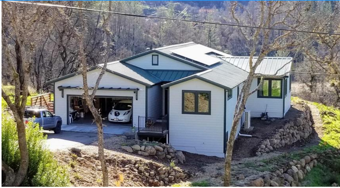
Hirsch residence: First SCP Advanced Energy Rebuild
