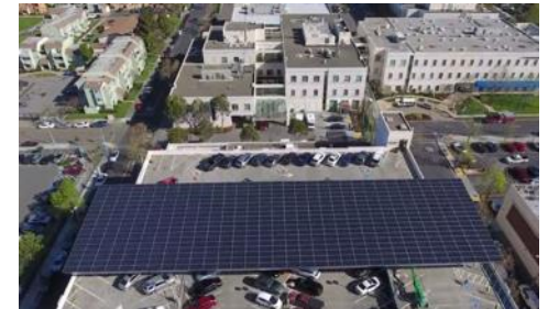
Kaiser Permanente Richmond microgrid
