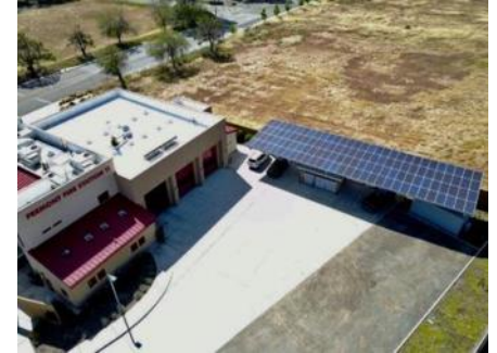
Fremont Fire Station microgrid
