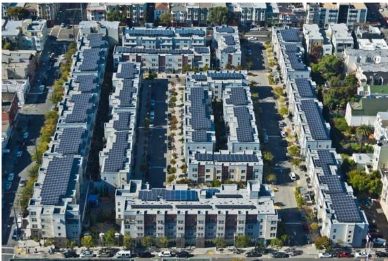
Valencia Gardens Energy Storage Project
