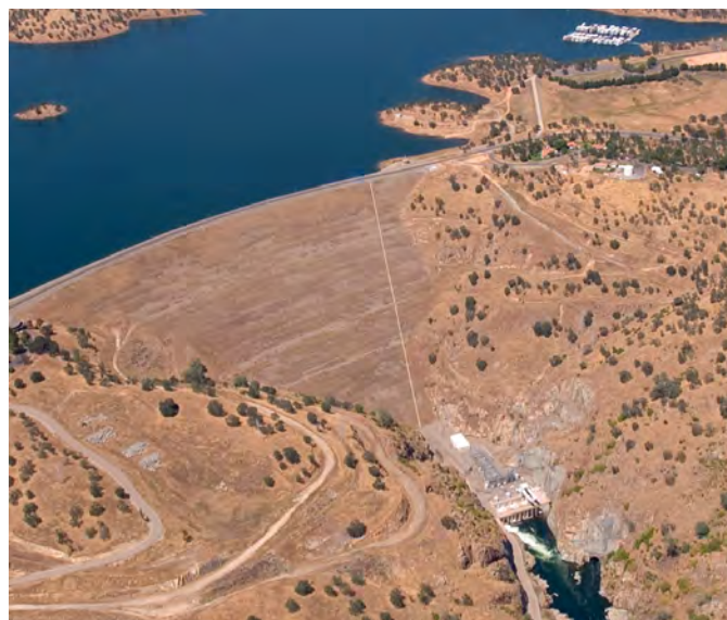
Don Pedro Dam and powerhouse. Photo: Turlock Irrigation District
