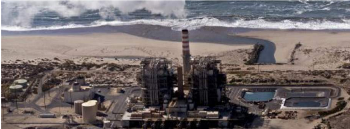
Puente Peaker Plant in Oxnard
