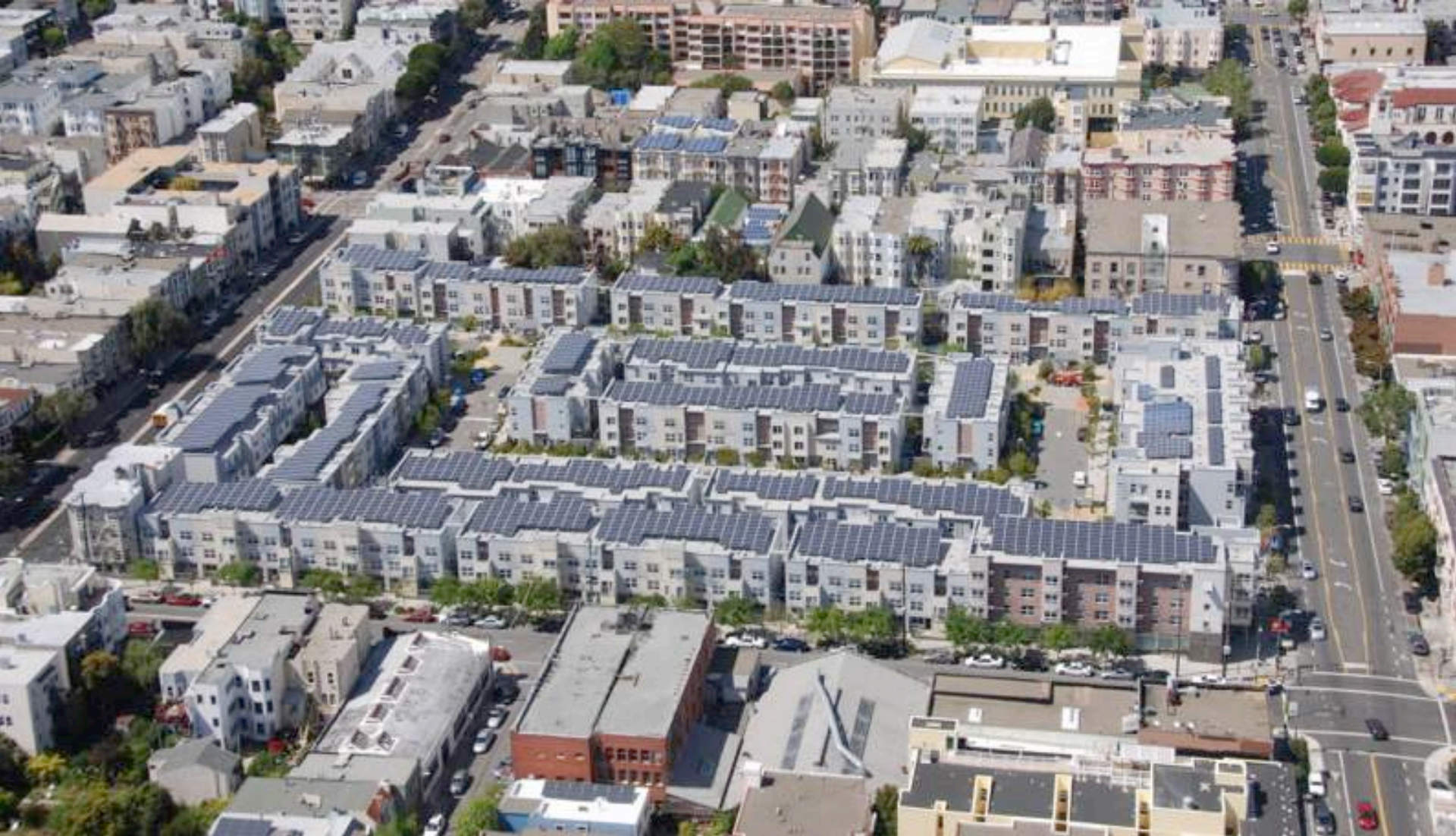
Ecoplexus WDG solar project at the Valencia Gardens Apartments in San Francisco, ~800 kW equivalent to ~80% of annual load.
