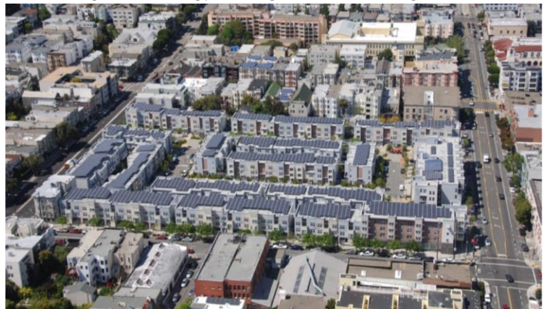
This project will deploy an optimized energy storage system to support the existing solar PV on top of the Valencia Gardens complex, pictured above. Photo credit: EcoPlexus.
