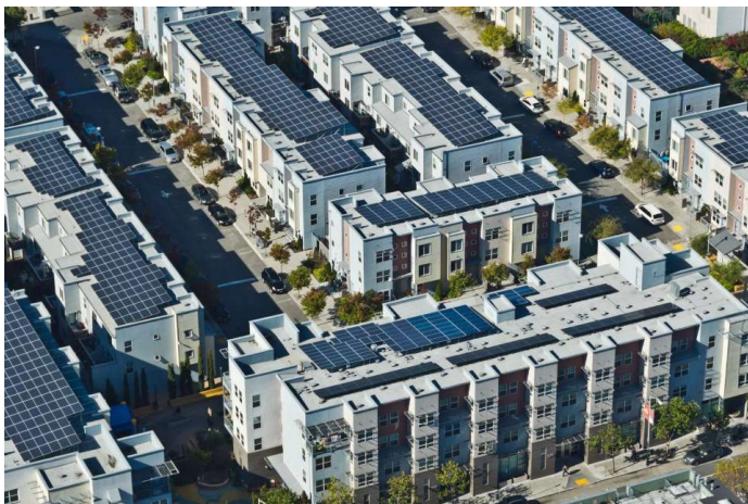
Valencia Gardens with existing solar
