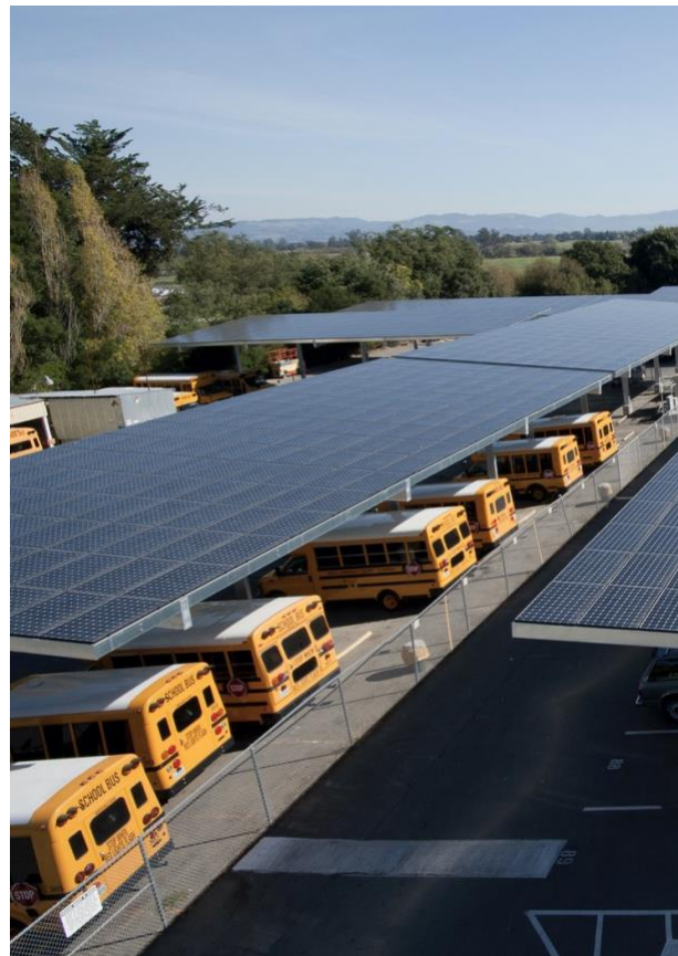
Solar parking canopies shading school buses at Analy High School, a Sage Energy site in the West Sonoma County Union High School District.
