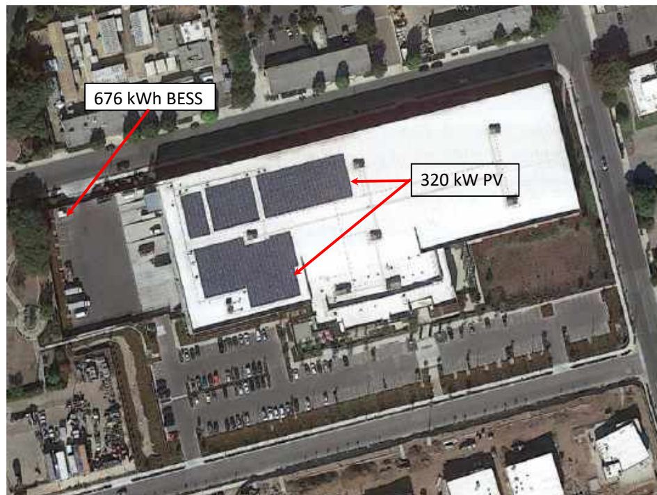
Direct Relief Solar Microgrid
