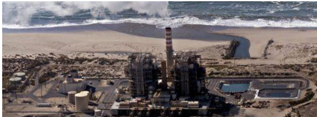
Puente Peaker Plant in Oxnard
