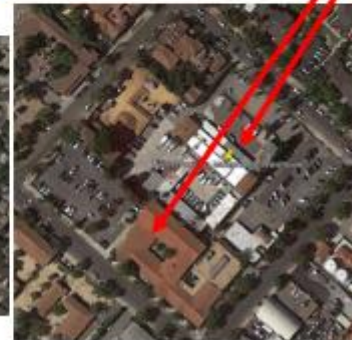
District Food Warehouse & District Office
