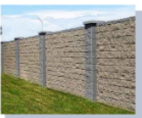
PERIMETER WALL CONCEPT - CMU 8' HEIGHT MATERIAL: MASONRY
