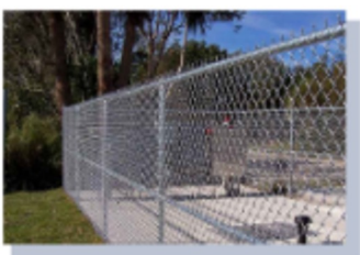
INTERIOR 6' TALL CHAIN-LINK SECURITY FENCE (AT EQUIPMENT AREA) MATERIAL: METAL
