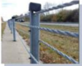
TENSION WIRE BARRIER (SAFETY RAIL FOR INTERIOR DRIVES)
