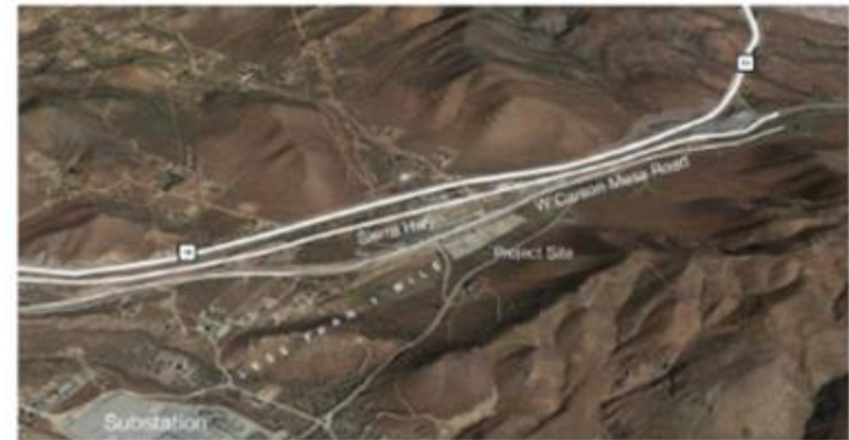
Adjacent to Grid Infrastructure
