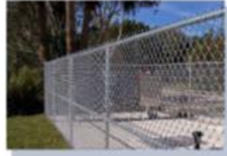
BARRIER 6' TALL CHAIN-LINK SECURITY FENCE (AT EQUIPMENT AREA)
