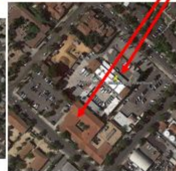
District Food Warehouse & District Office
